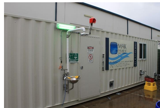
Containerised WTP with access door, window and safety shower & eyewash station
