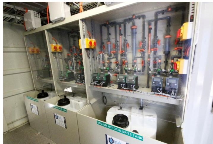
Acid, caustic and sodium hypochlorite dosing systems
