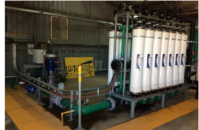
MAK Skid Mounted 1,500 m 3 /day UF Plant
