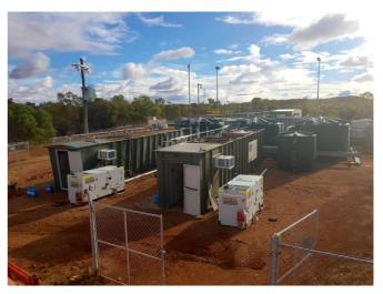
Activated Sludge Bioreactor (ASBR) on site in Queensland
