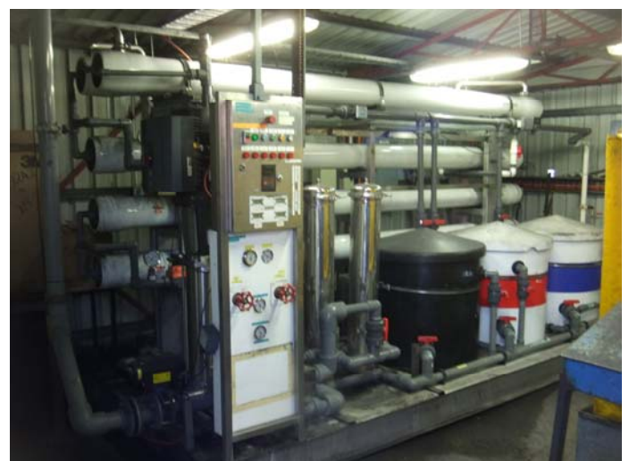
A third reverse osmosis stage was added to increase the recovery and reduce the brine volume
