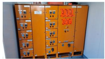
Form-4 mine-spec control panel to client specifications
