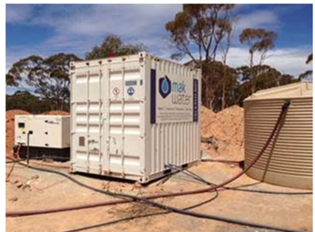
The Brackish Water Reverse Osmosis plant on site in the Goldfields
