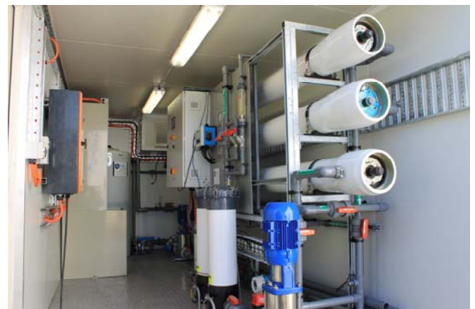
The completed brackish water reverse osmosis plant
