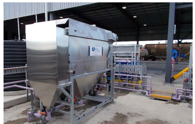
The dissolved air flotation system on site in Hexham, NSW
