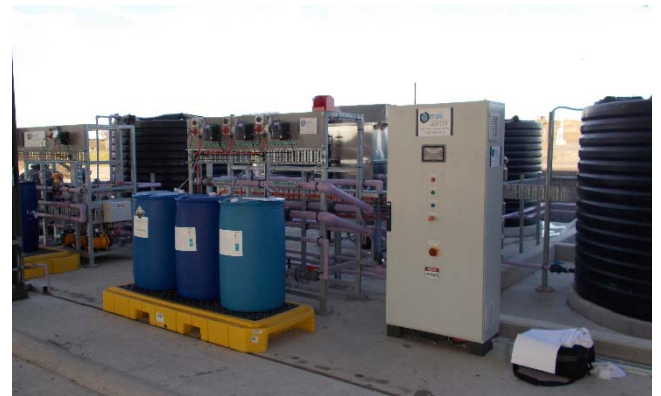
The DAF system includes post-clarification multimedia filtration, pH neutralisation, ultraviolet sterilisation and chlorine dosing
