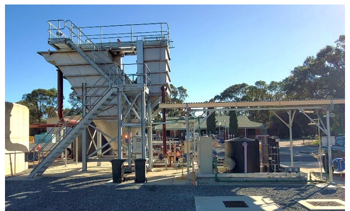
MAK Water custom Lamella Clarifier installed onsite
