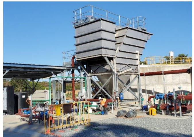
MAK Water custom Lamella Clarifier installed onsite
