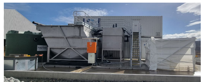
Lamella clarifier next to stacked containers
