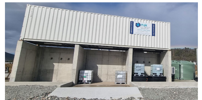
Filter Press container mounted atop a concrete bund for dewatered cake collection & storage
