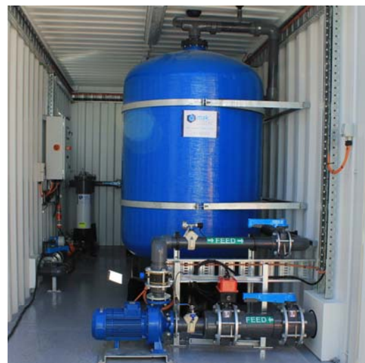
Containerised MMF plant capable of treating 1,000 m 3 per day
